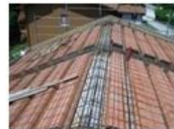
COPERTURE IN LATERO-CEMENTO
